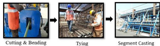
Figure 1. Segmental Production Process
